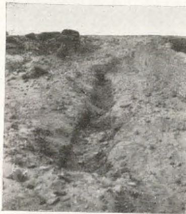
1. — Water supply pipe in a street at Philadelphia.
